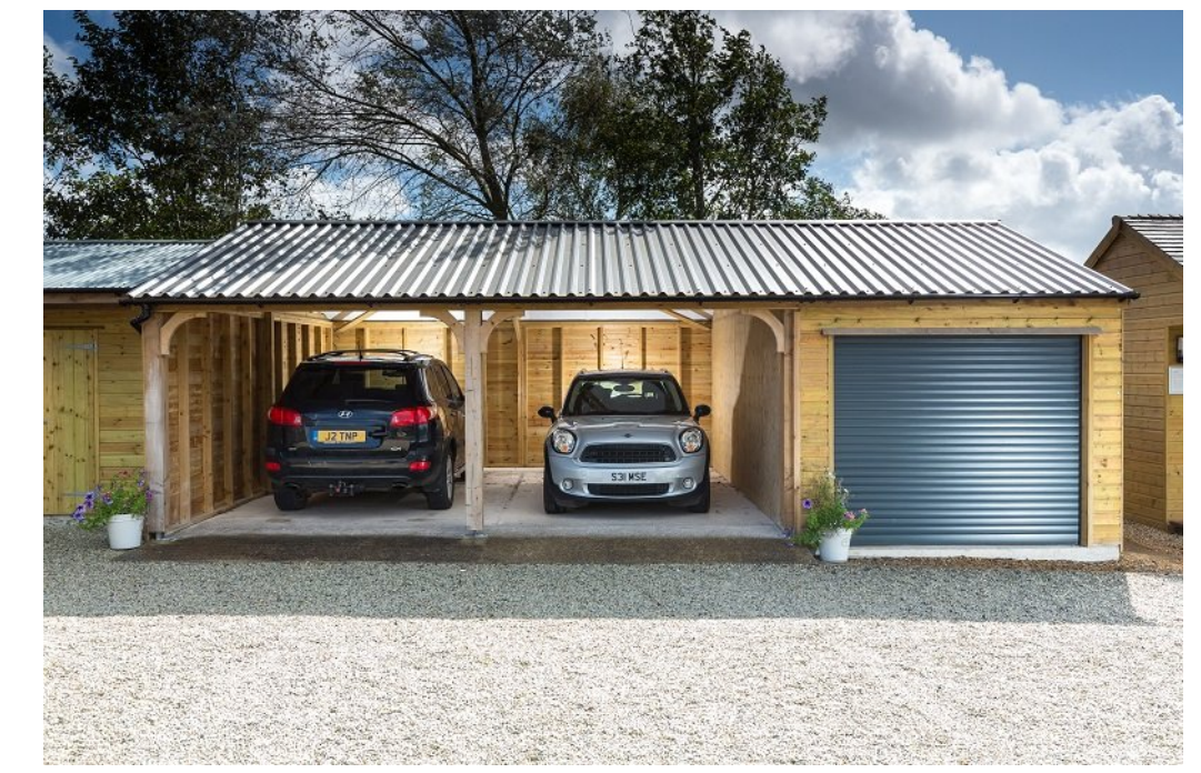
Cladco Metal sheet roofing
